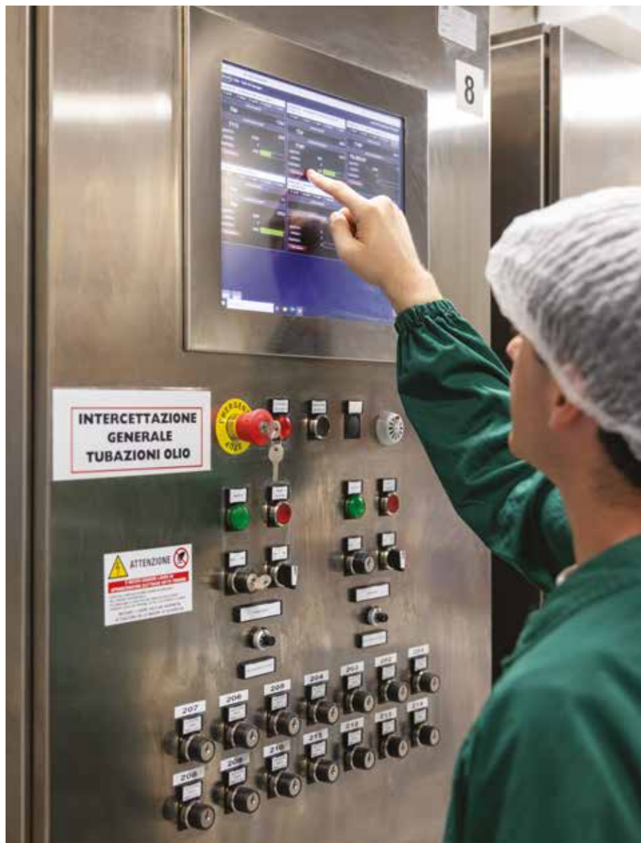
An integrated management and control system for oil discharge, storage and handling of bulk/unbottled oil
